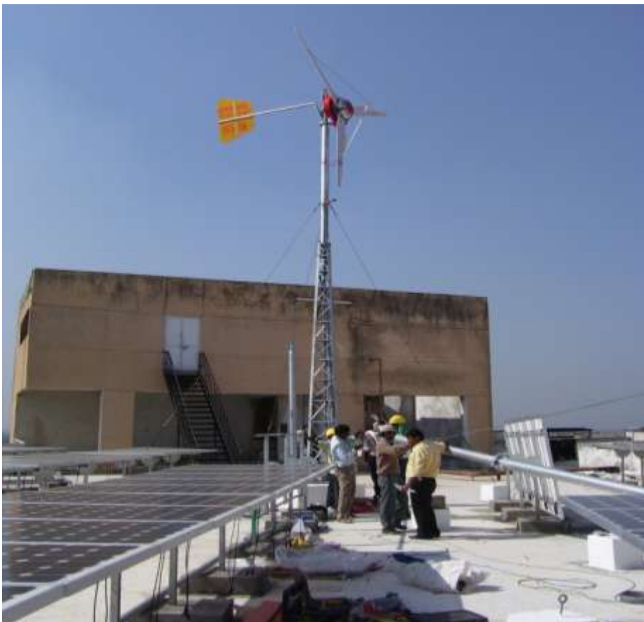
10 KW Wind-Solar Hybrid system installed at Udyog Bhavan roof-top
